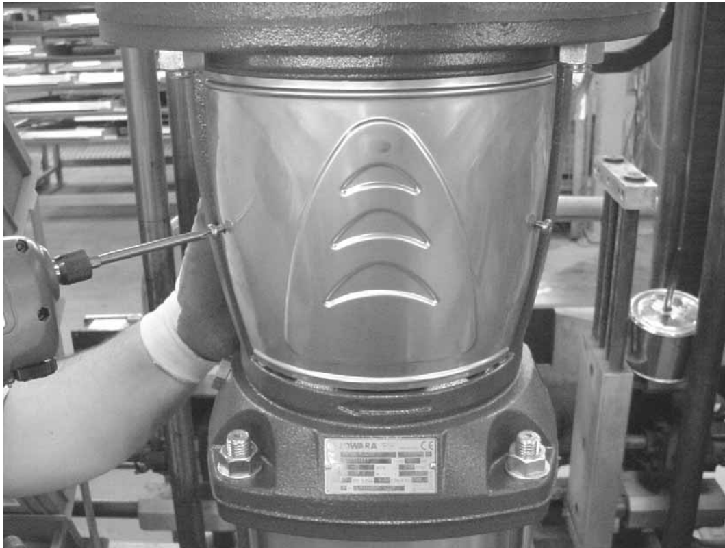
Removal of coupling guard
