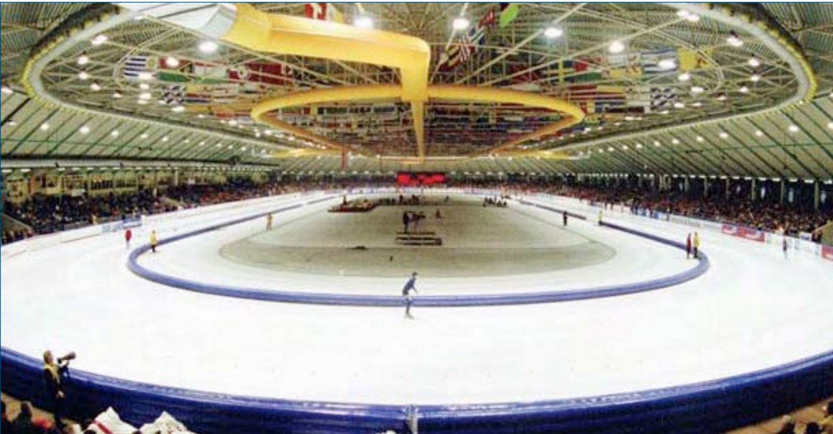
Thialf ice skating track complex in Heereveen, The Netherlands.
